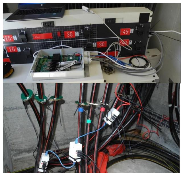
**Figure 4.** GridBox installation in a transformer station (BKW).
